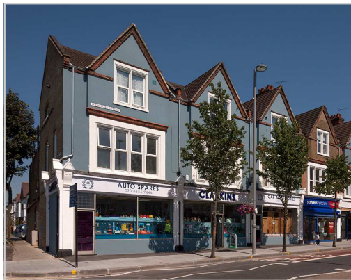
Left: This shop extends across three units, but the fascia sign is broken into sections rather than extending across the whole shop front.
